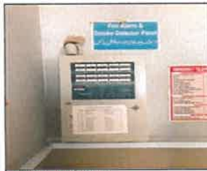
Photo of fire safety equipment Smoke detector and fire alarm panel.JPG
